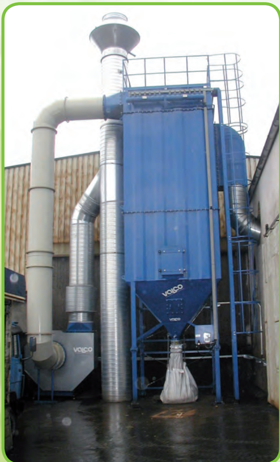
▼ Dust extraction system with bag filters for 40,000 m 3 /h, cast steel foundry
