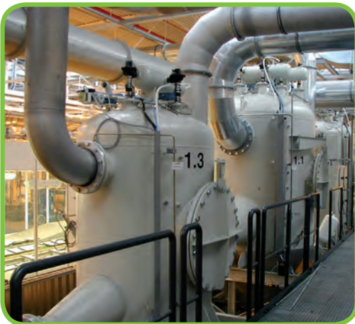
ATEX-cartridge filter, 11 bar pressure-resistant for explosive powder
