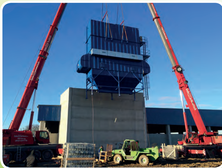
Bag filter system for 175,000 m 3 /h, 36 tons system weight
