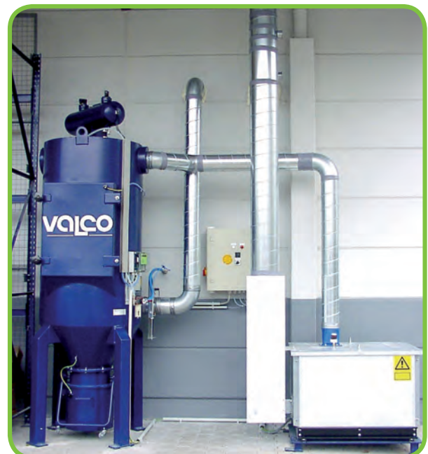
▼ Central high vacuum extraction- and filter system, 2000 m 3 /h, 20kPa, 22 kW, for extraction of welding dust at the torch
