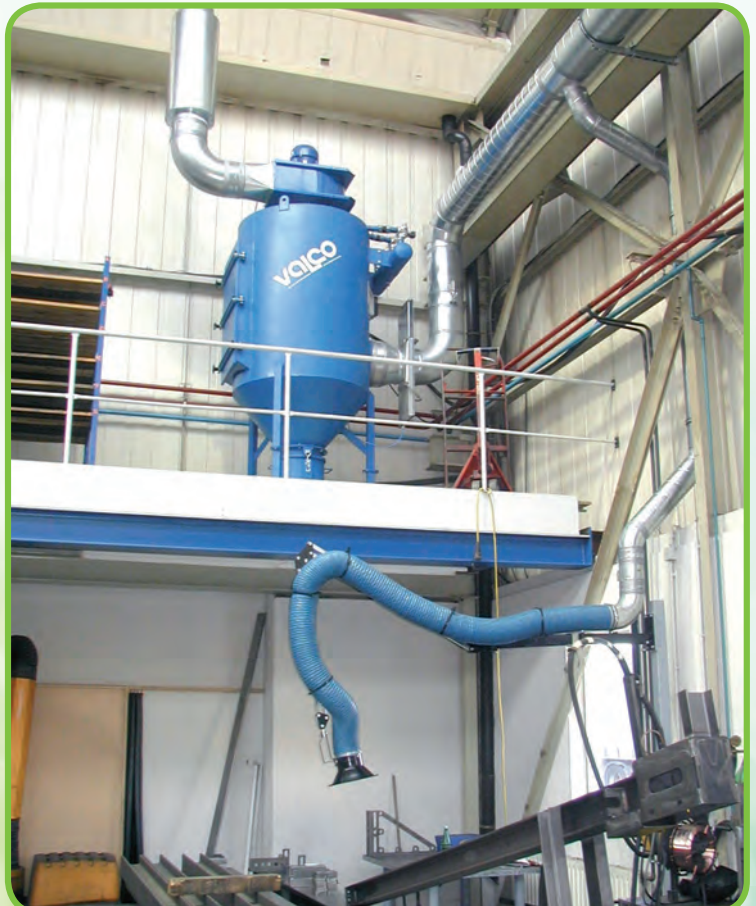
▼ Compact filter system type RX-7500 for welding fume extraction via extraction arms.
